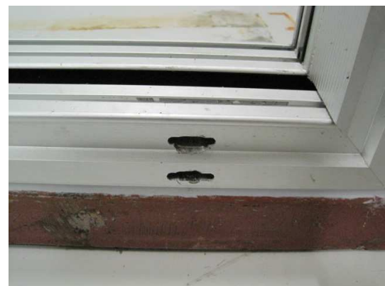
Picture Rebate drainage 1, to outside front
