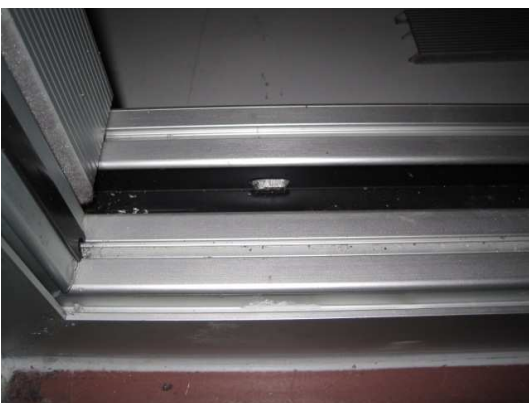
Picture Rebate drainage 1, inside rebate
